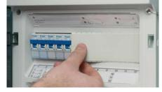
Additional space with DIN rail over the total enclosure width for electrical devices not to be manually actuated. Installation depth 72 mm. Installation height max. 125 mm resp. 150 mm.
