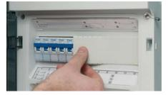
12 to 54 modules: attached blanking strips for DIN rail equipment openings
